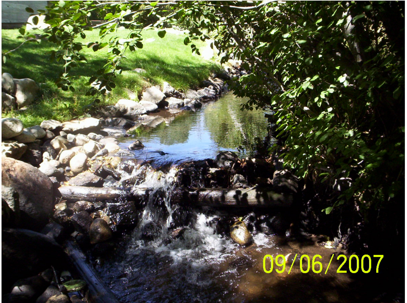
Figure B-6. One example of instream rock dams constructed in Reach B of Mammoth Creek. Some of the instream rock dams are substantial, and may have the potential to act as a fish barrier under low flow conditions.
