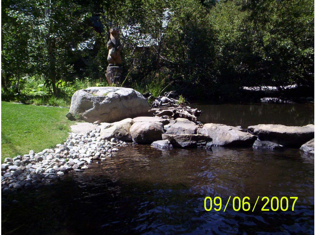
Figure B-7. One example of a private parcel exhibiting grass installation up to the creek bank, rocks installed along the creek bank, and an instream rock dam.
