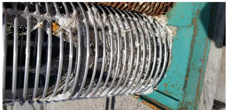
This is a picture of the influent grinder completing clogged with wipes. The District spent over \$200,000 to replace the grinder with a trash removal system due to the persistent problems cause by the influx of wipes at the wastewater treatment plant.
