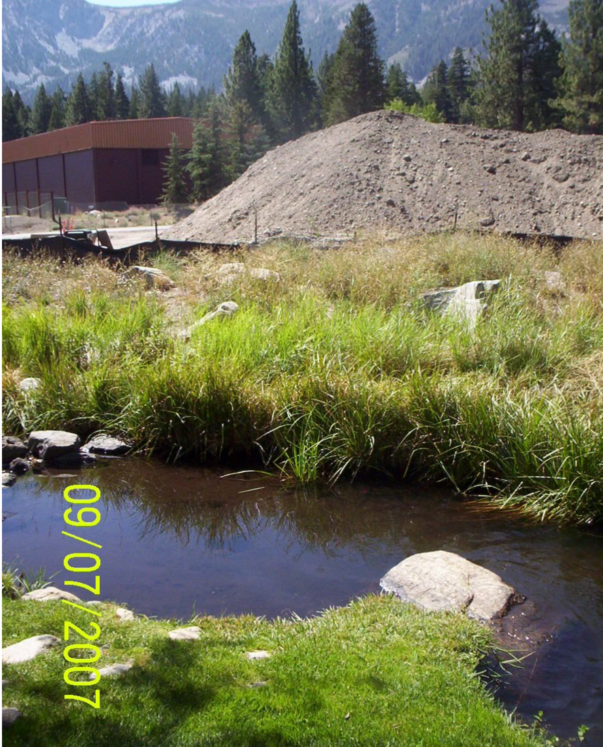
Figure B-3. Ongoing development across Mammoth Creek from Snowcreek IV, near MCWD's groundwater treatment plant.
